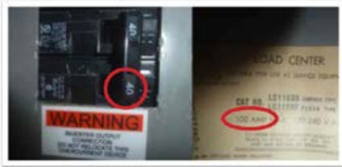
Photo 2: Backfed PV breaker not installed at opposite end of buss bar from main breaker: 2014 NEC690.12(D)(2)(3)(b)
